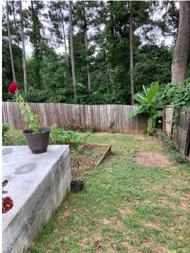
Concrete Slab at Finished Floor Elevation (Side)
