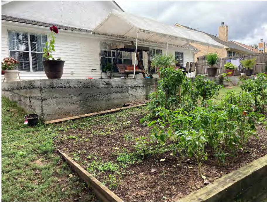
Concrete Slab at Finished Floor Elevation (Front)
