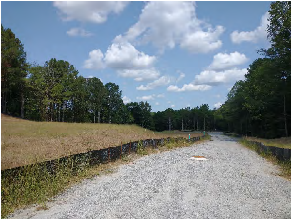
View from Private Drive towards rear of property
